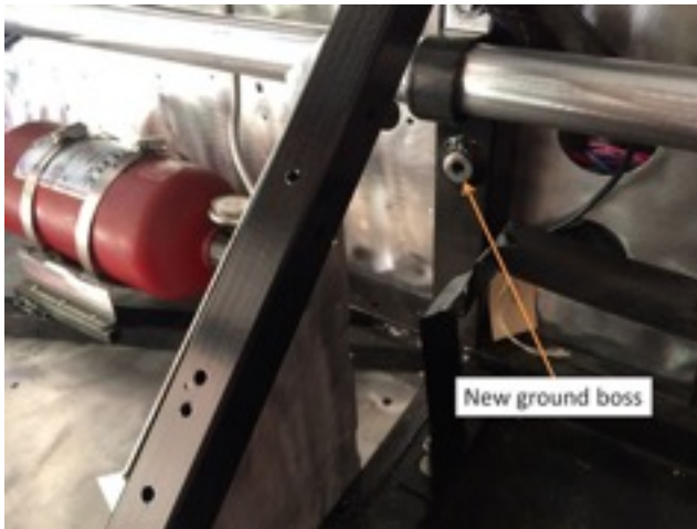
Figure 6 – Ground Boss #1 location
