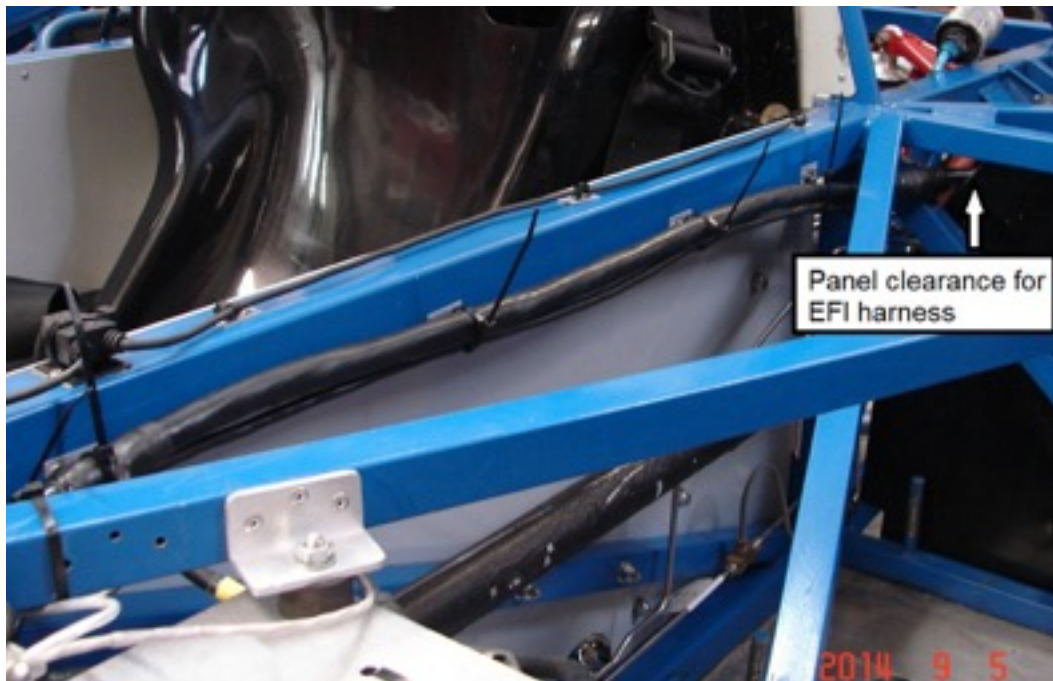
Figure 16 – EFI Harness Installed (Part 1)
